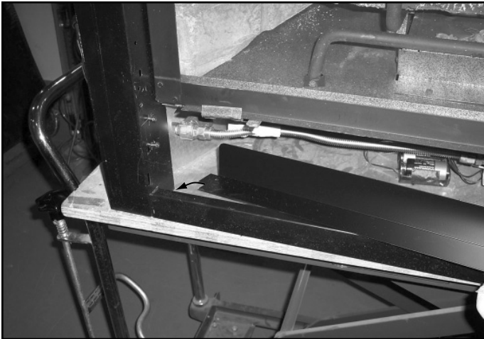
Figure 14.13 Installing Floor Cover
